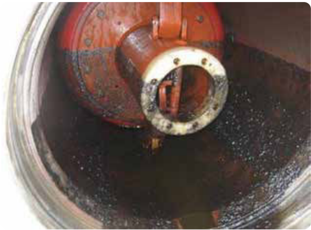
Figure 1. Result of pigging a “dry” network
